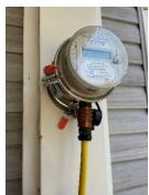
The easiest method is with a GenerLink™ (https://generlink.ca/). It is an approved device that goes between the meter and the meter base on your home, allowing a generator to be plugged in.
