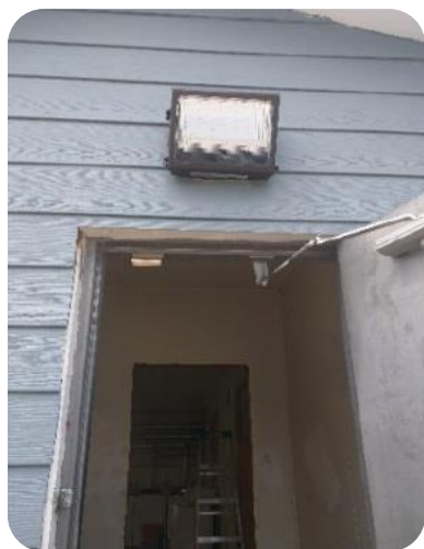
Figure 2 - LED wallpack installed above a door
