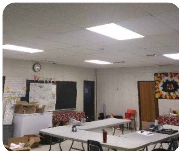
Figure 1 – New LED lights installed in a Kingfisher Lake First Nation building through the Commercial Lighting Program
