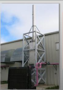
EXHAUST SYSTEM: Engine exhaust is released into the atmosphere through mufflers and exhaust stacks. Strick emission and noise regulations are put in place to minimize noise and pollutants.
